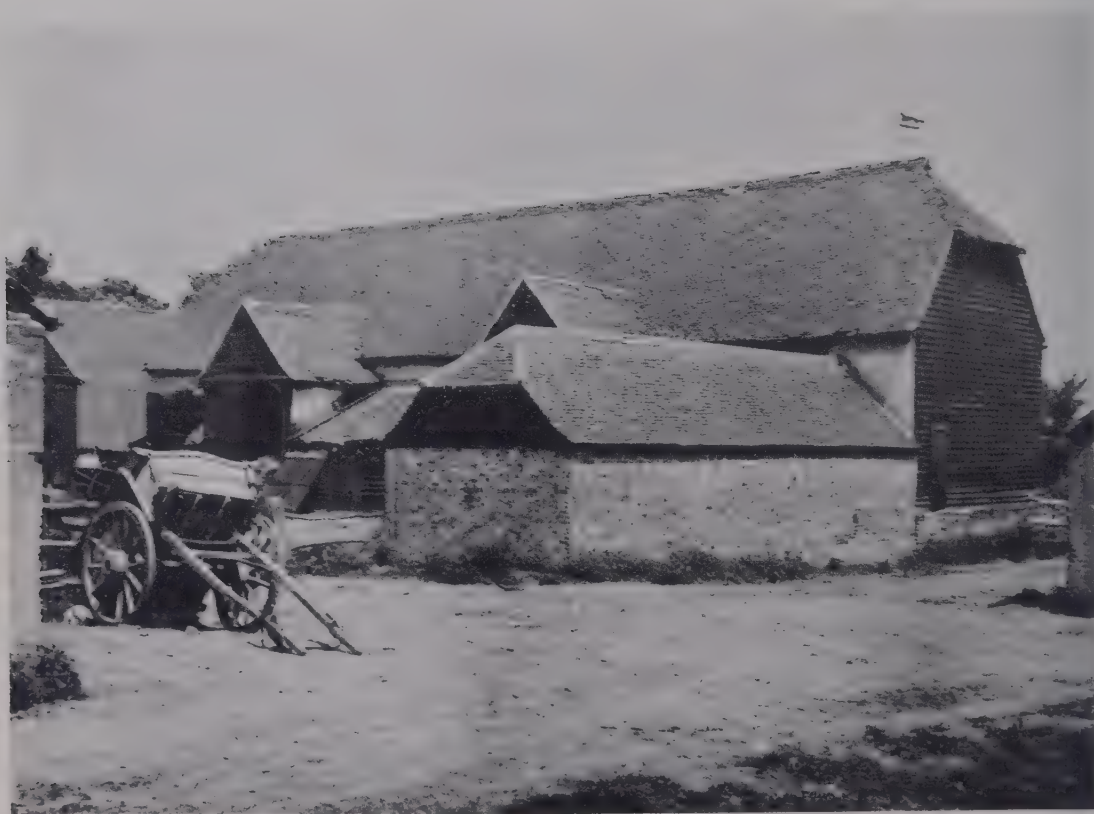
BARNS AT ROOKWOOD HALL, ABBESS RODING
