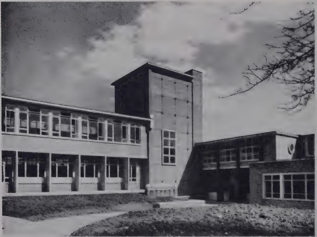
LUCTON SECONDARY MODERN SCHOOL, DEBDEN Built 1950
