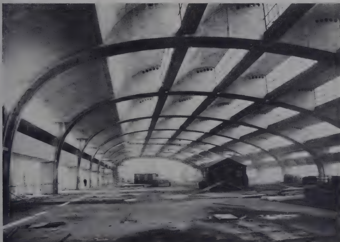
Bank of England Printing Works: Interior of Main Hall under construction, 1954
