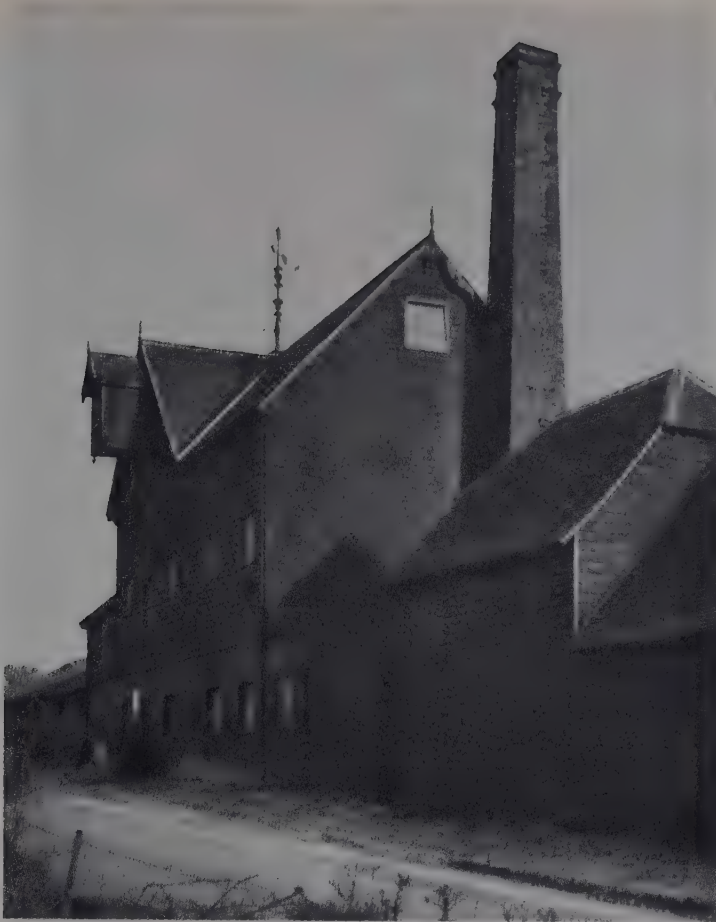
FORMER STEAM MILL, NAVESTOCK
