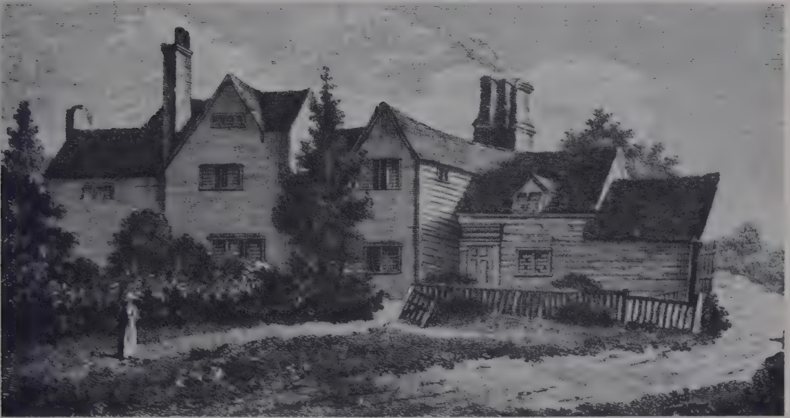
THE FORMER RECTORY, STONDON MASSEY Built in the early 17th century, demolished c. 1800
