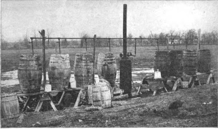
a. Barnes Bros. plant for boiling the lime, sulphur and salt mixture.
