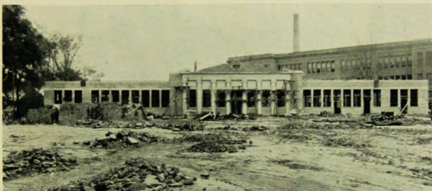
Cafeteria Building in Construction
