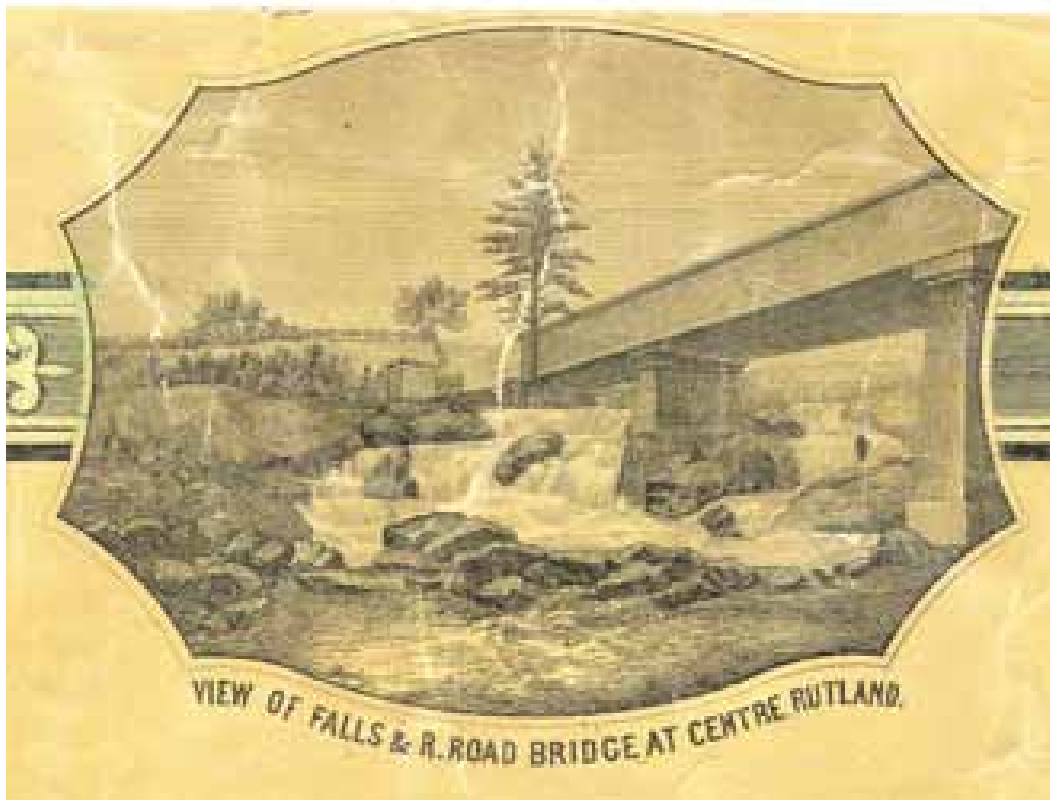
View of Falls & R.Road Bridge Rutland
